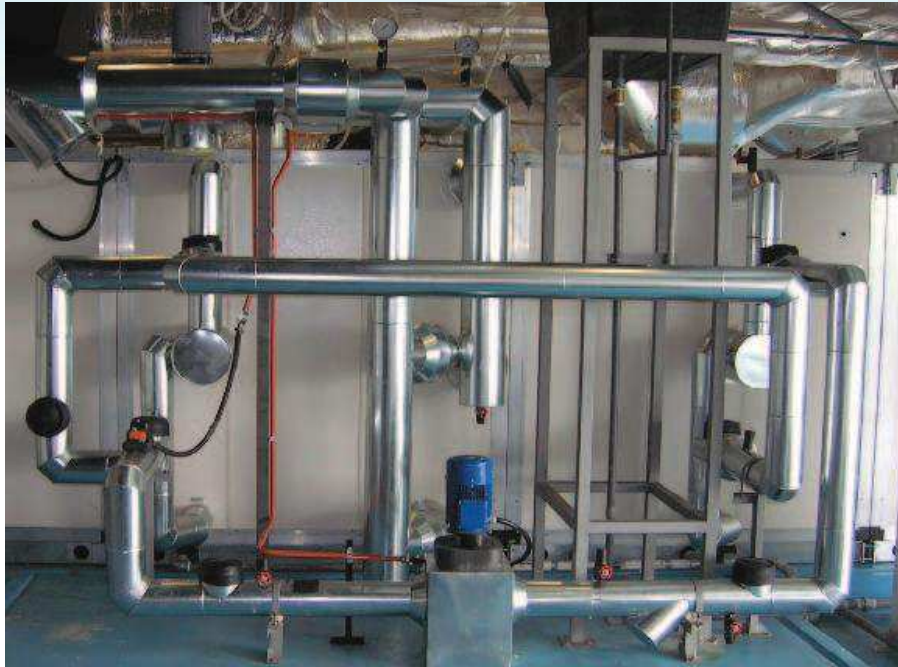
Jobsite piping connection of Coil Loop
